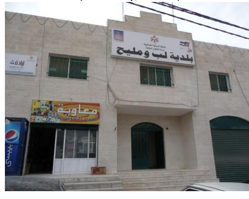
Figure 4 City-hall with 4 Small Shops at the Ground Floor (Maan city, Jordan)
