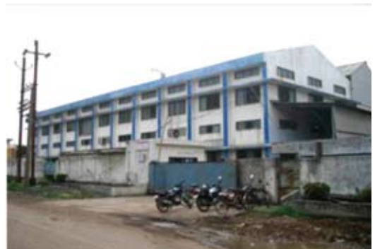
Plant buildings with gates and guard post
