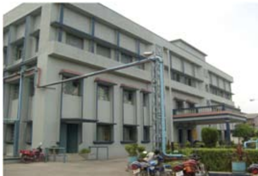
Front entrance to the main building
