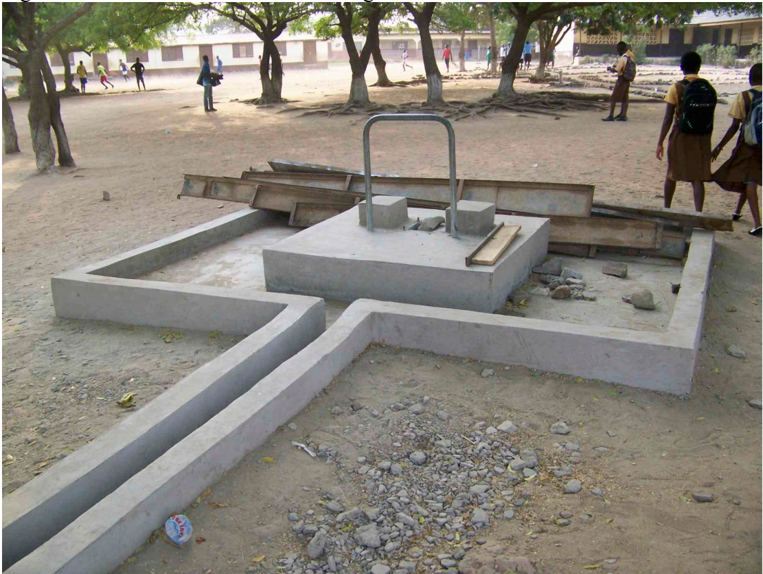
Figure A7: Borehole at a School – In Progress
