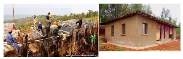
In South African, MMA Architects have even created two-story houses using earth bags inside wooden and steel frames. Thus, the material can be robust, and is often much cheaper than fired brick.
