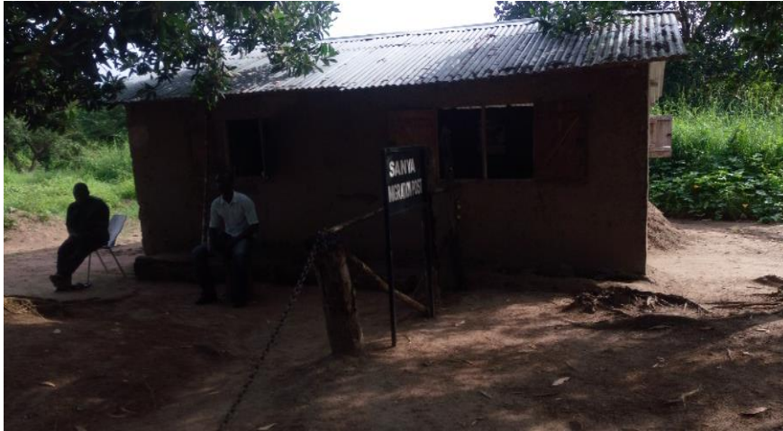
Photo of dilapidated Sanya Post
