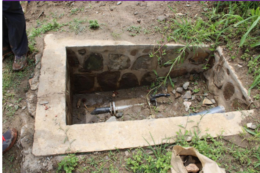
Figure 2: Example maintenance issue for the irrigation infrastructure
