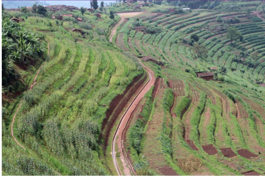
Figure 1: Primary canal in one of the studied hillside irrigation sites, Karongi District
