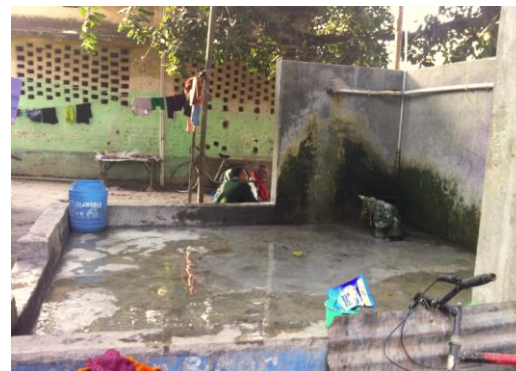
Figure 4 Open bathing facilities -Ambedkar Bhawan, Nala Road
