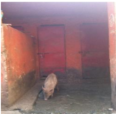
Figure 3 Abandoned toilets- Ambedkar Bhawan, Nala Road
