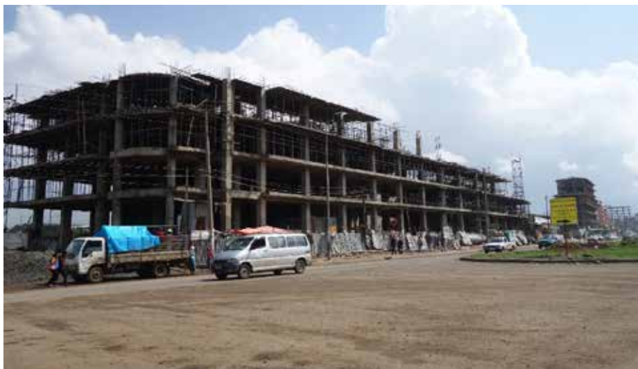
Construction along new roads in Addis Ababa (Source: Bird and Franklin, 2015)
