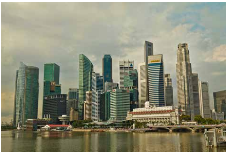
High density central business district in Singapore (Source: Van den Broek, Flickr)
