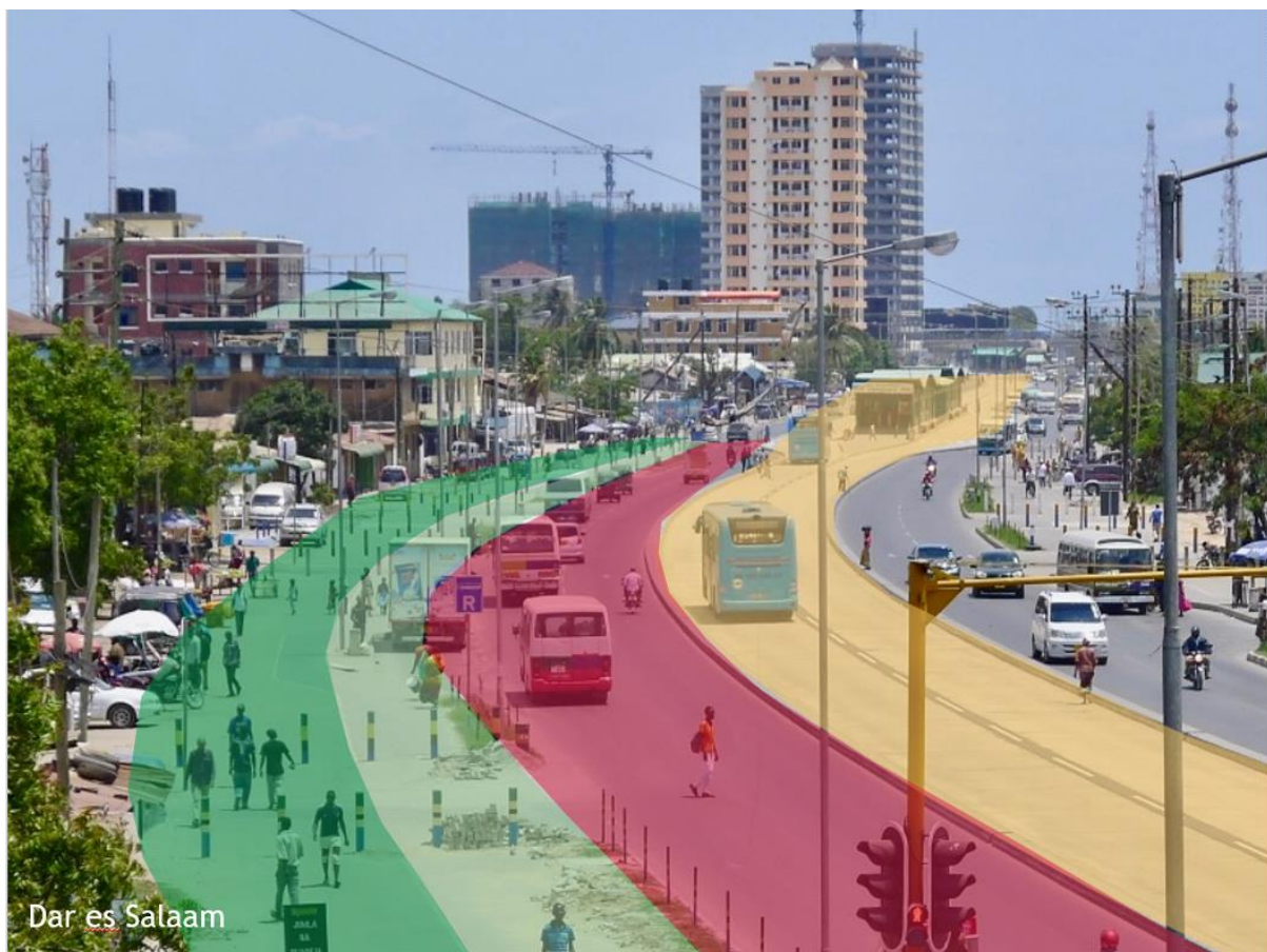
Figure 6: Complete street in Dar es Salaam
