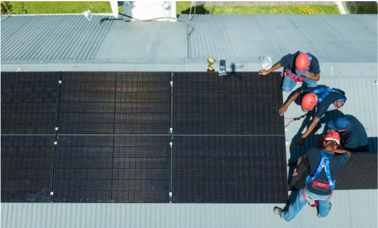
Workers install solar panels on the roof of a house in South Africa. Photo by Getty Images.
