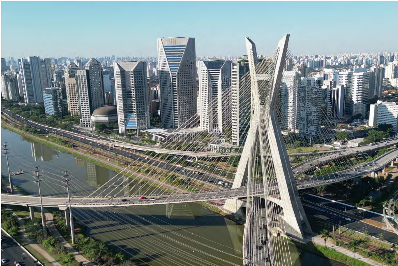
Figure 6: Estaiada Bridge (UOAE)
