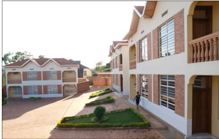
Land used for schools are often exempted - School in Kigali, Rwanda (Photograph: Brian Dolinger)
